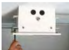
Adjust to ensure ceiling integrity
