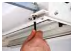
Single screw height adjustment
