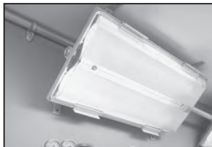
The FVS is rated for Zone 1 and Simultaneous Presence.
