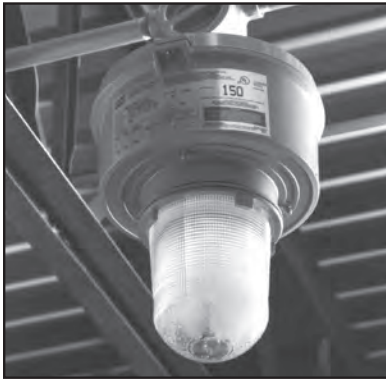
Champ® restricted breathing luminaires are rated Ex nR for Zone 2 areas.
