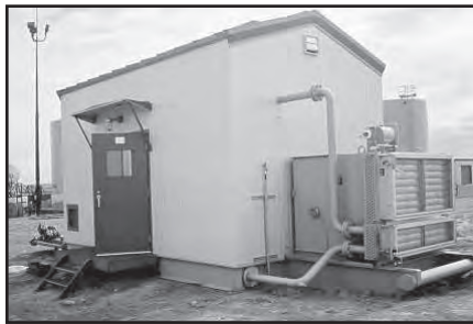
Remote Class I buildings that are not remotely monitored to ensure Zone 2 conditions can be met are classified Zone 1.
